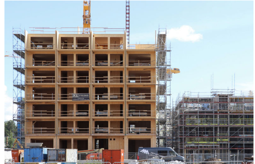
Kajstaden Tall Timber Building - CF Møller Architects
